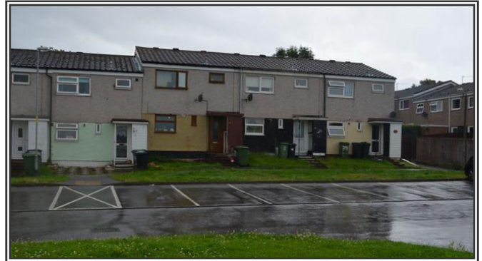
Properties in Woodrow prior to completion of external wall insulation works.
